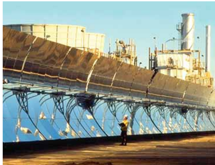
Parabolic mirrors focus the sun's energy on a small area, generating heat, which can then be converted to electricity. Large-scale solar troughs, like these in California, have tremendous commercial energy potential.
