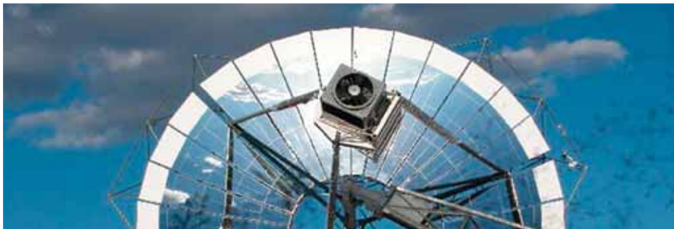
A dish system collects energy from the sun and concentrates it, producing heat that is transferred to a generator.
