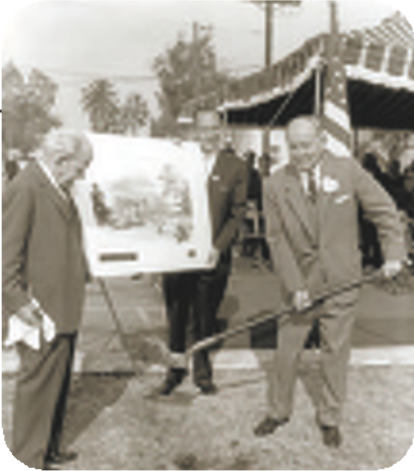
Olin Hall groundbreaking
